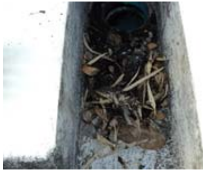
leaves block the water drainage
